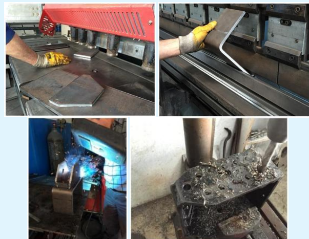
Figure 8: Cutting, forming, welding and drilling of steel plate.
