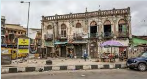
Figure 2: The state of Ilojo Bar before demolition.
