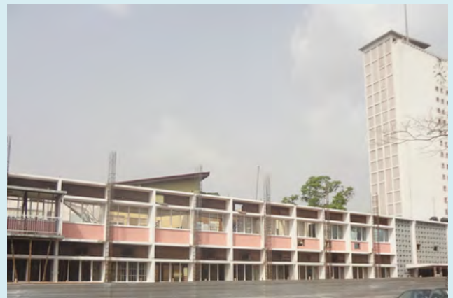
Figure 3: University of Ibadan Central Administration Building during modification.
