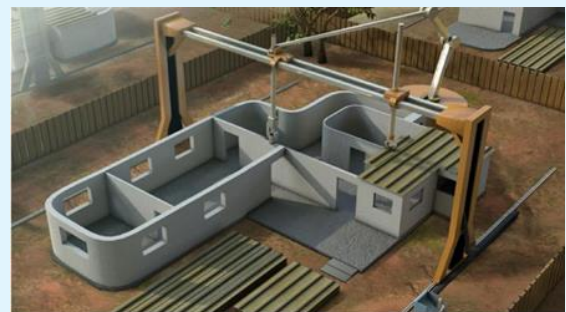
Figure 10: 3d printed house, Counter Crafting.
