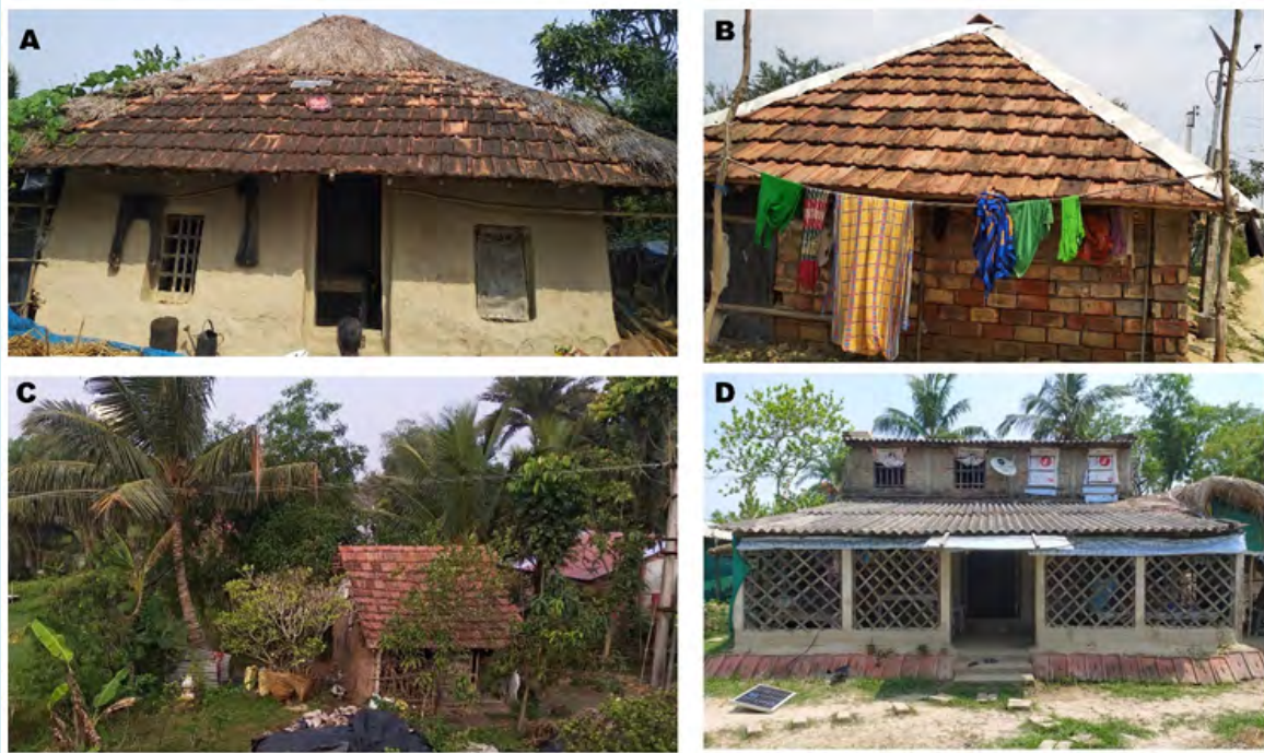
Figure 2: Structure of rural and semi-urban dwellings unit (A) used the tailed (tali) as roof materials and clay as wall materials; (B) used tailed (tali) as roof materials and fired brick as wall materials; (C) green area in the surrounding environment; (D) windows pattern.
