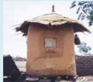
Figure 2: Basket mudded wall storage structure
