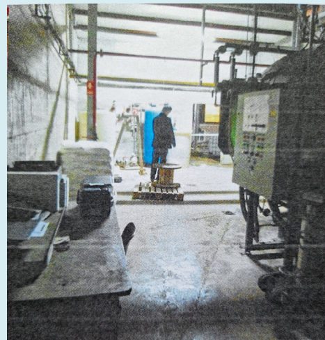
Figure 3: Overall view of the hanging scene.
