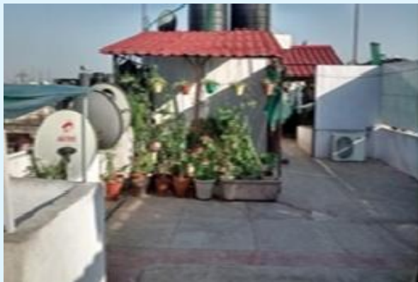
Figure 3: Terrace repaired and cottages made.
