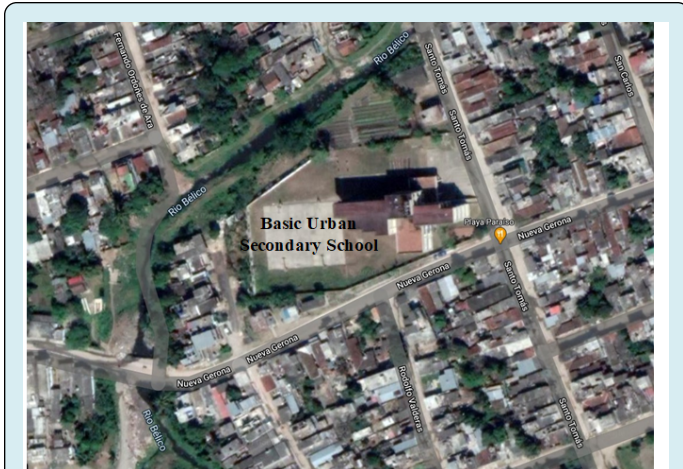
Figure 2: Satellite photo, where the “Antonio Aucar Jimenez” Basic Urban Secondary School is observed. Very close to the school runs the Belico river whose waters are murky, dirty and with high levels of contamination.
