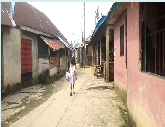
Plate 3: A View of an Access Road without Drainage.
