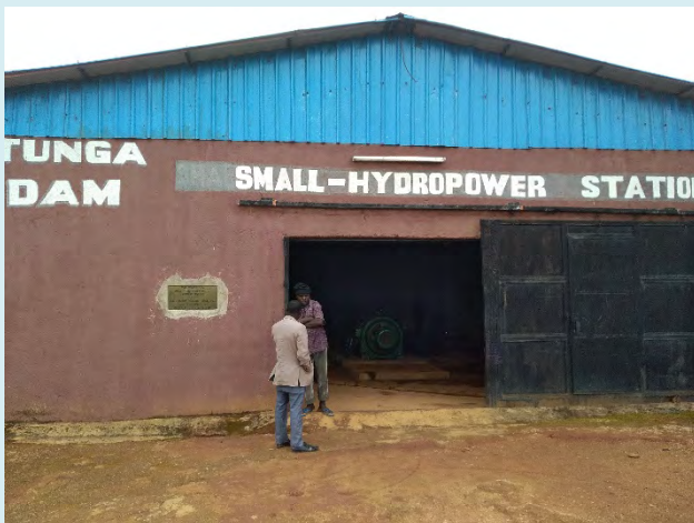
Plate 1: Tunga Small Hydropower dam.
