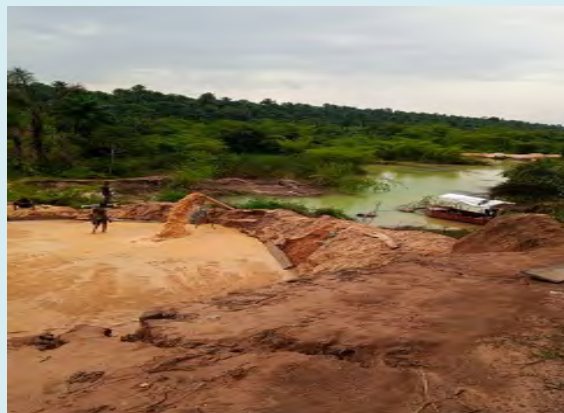
Plate 4: Dredgers drilling Sand in Commercial Quantities to meet demand.
