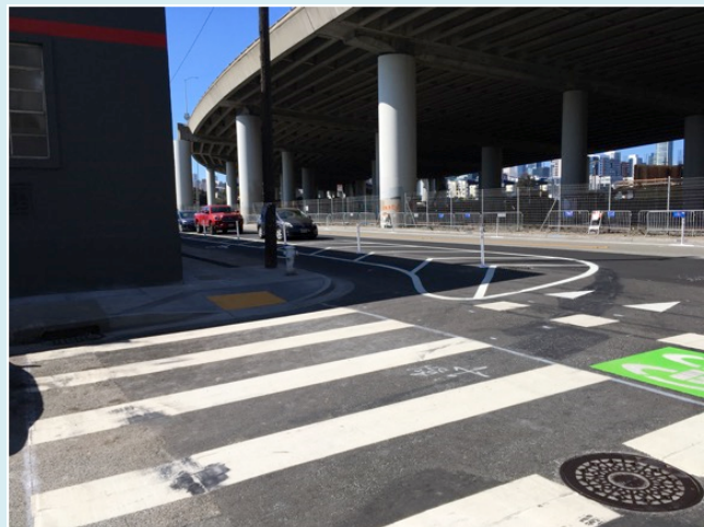
Figure 8: View of same intersection as in Figure 7 showing not only blocked view of oncoming traffic on 7th but also how traffic on oncoming lane cannot see bicycle riders in lane hidden by cars.
