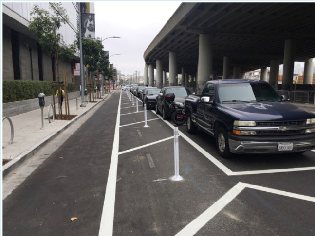
Figure 4: View of bike lane designed to prevent car door opening to injure or impede bicyclists. Parking spaces are now in what was a traffic lane with traffic moving passed parked cars in only lane left.
