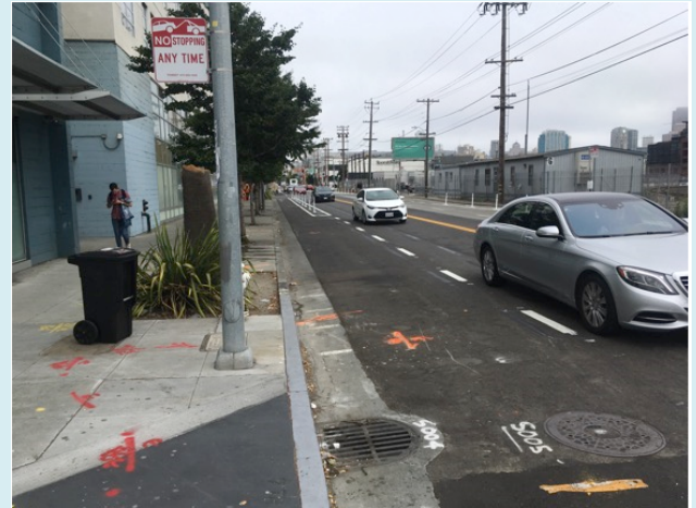
Figure 5: View of 7th Street farther north of previous images showing loss of parking and bike lanes. Street has been engineered to remove as much parking as possible and provide space for “safe” lanes for bikes. Traffic is squeezed into one lane in each direction. Design creates an opportunity for drivers to enter the bike lane to attempt to pass stopped traffic creating dangerous conditions.
