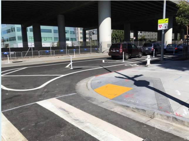
Figure 7: View of intersection with stop sign where drivers' view of oncoming traffic is blocked by parked cars in former curb lane.
