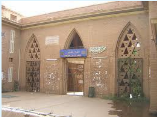
Figure 3: Red bricks hollow walls, buildings.
