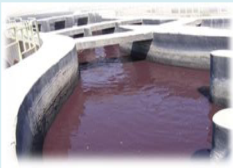
Figure 1: Contamination of wastewater ponds at 10 th of Ramadan industrial city – Sharqia Governorate - Egypt with textile red dyes (with permission of Ewida, et al. [48]).
