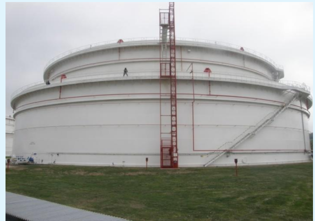
Figure 2: Storage tank with volume of 70,000 m 3 .
