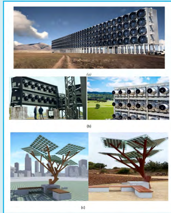
Figure 44: The typical large-scale direct air capture plants modular system by Carbon Engineering USA and Climeworks in Switzerland [28, 29].
