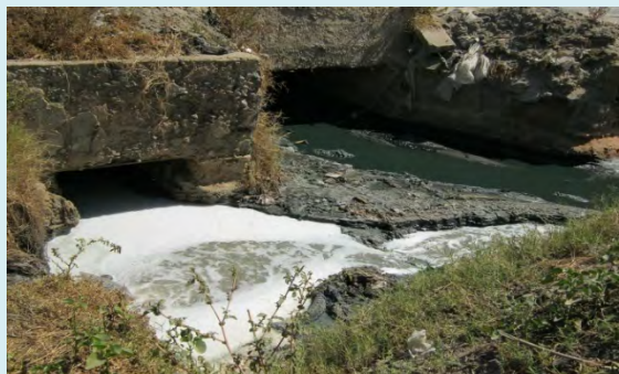
Figure 2: Effluent Discharge Point, MARIO JOSE Tanning Company.
